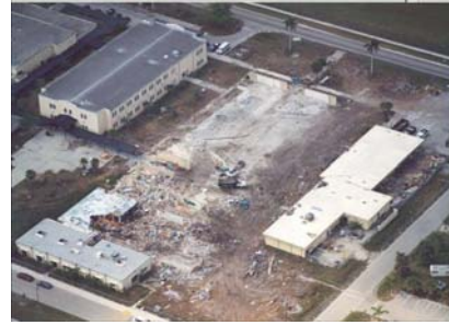
Charlotte High School - Hurricane Charley - August 2004 Charlotte County Public Schools, Florida Modular City Report
